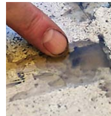
Wall of porous travertine in Kamppi (= the Kamppi Terminal and Shopping Center), Helsinki.
