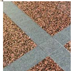
Reconstructed floor of the Helsinki Main Railway Station. Gray rock = fine-grained Kuru granite, red = coarse-grained Taivassalo rapakivi granite.
